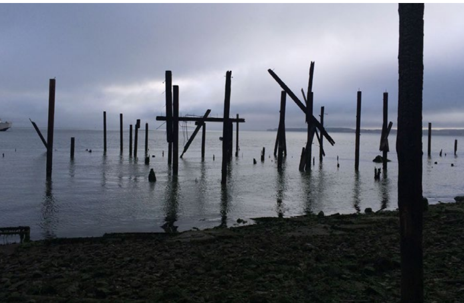
Creosote-treated pilings at the Red Rocks warehouse site in Richmond. Photo by Marilyn Latta, State Coastal Conservancy.
